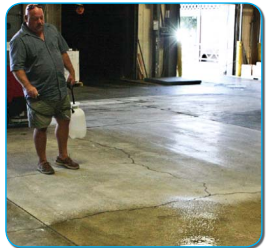
FIGURE 5-A: LAYING DOWN DENSIFIER WITH SPRAY TOOL.
