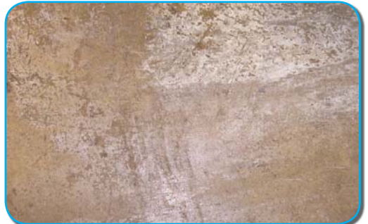
FIGURE 5-B: LEAVING DENSIFIER ON THE FLOOR TOO LONG CAN CAUSE DISCOLORIZATION.
