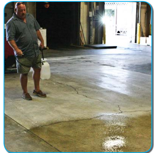
FIGURE 3-B: LAYING DOWN DENSIFIER WITH SPRAY TOOL.
