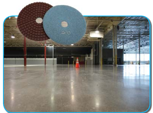
FIGURE 5-C: 400 GRIT BLUE SNAP! DISKS AND IMAGE OF FLOOR AFTER 400 GRIT DISKS.
