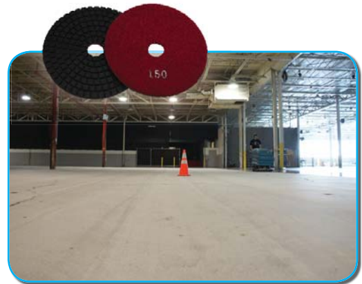
FIGURE 4-B: 150 GRIT GREEN SNAP! DIAMOND DISKS AND FLOOR AFTER 150 GRIT DISKS.
