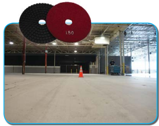
FIGURE 3-A: 150 GRIT GREEN SNAP! DIAMOND DISKS AND IMAGE OF FLOOR AFTER 150 GRIT DISKS.
