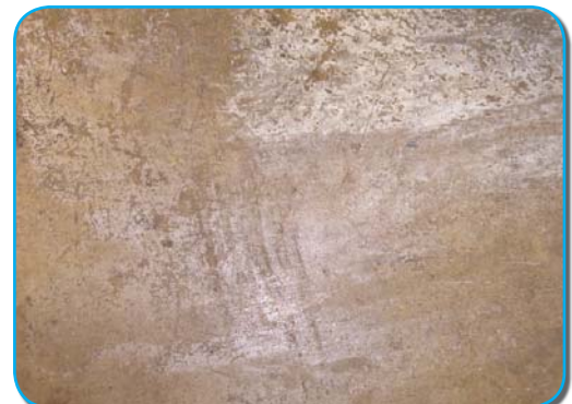
FIGURE 3-C: LEAVING DENSIFIER ON THE FLOOR TOO LONG CAN CAUSE DISCOLORIZATION.
